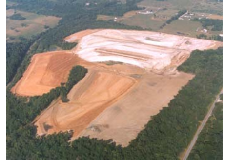
Gypsum Stacks Reclamation
