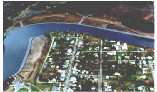
Containment of PCB Impacted Sediments
