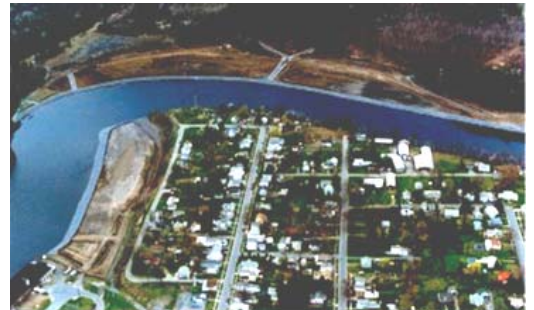
Containment of PCB Impacted Sediments
