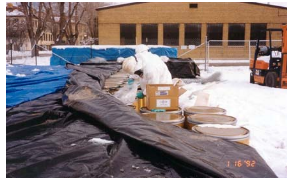
Drummed Waste Characterization For Off-Site Transport/Incineration/Disposal
