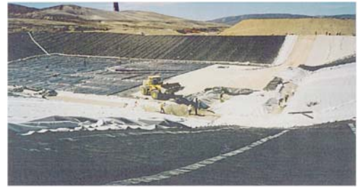
Arbiter Repository Construction
