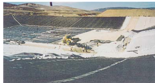
Arbiter Repository Construction
