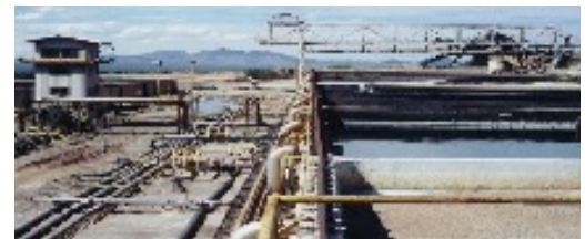
Leach Vats Demolition Cost Estimate
